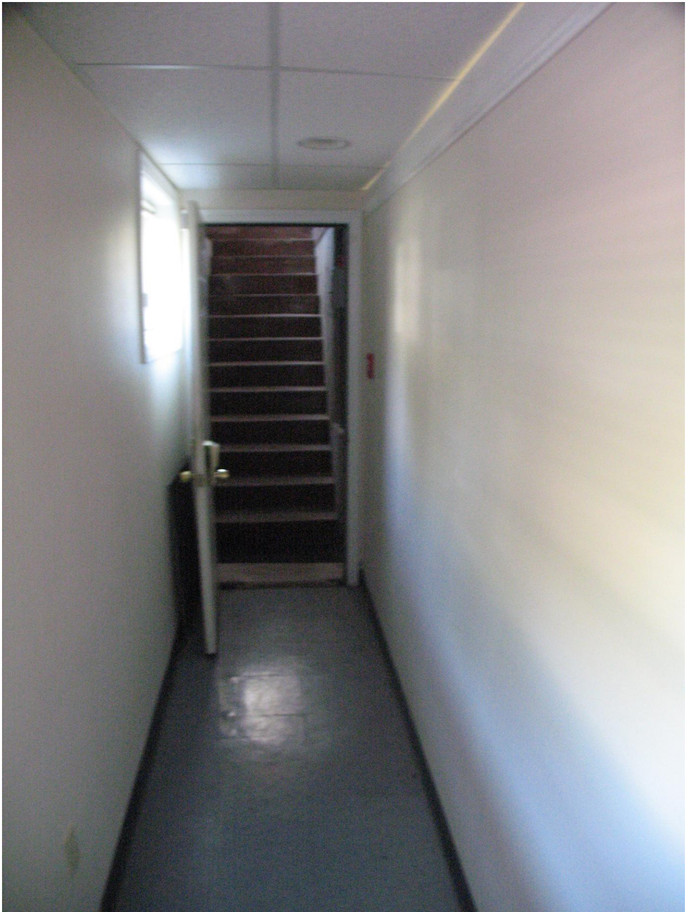
Figure 18: Rear egress stairway, below minimum standards
