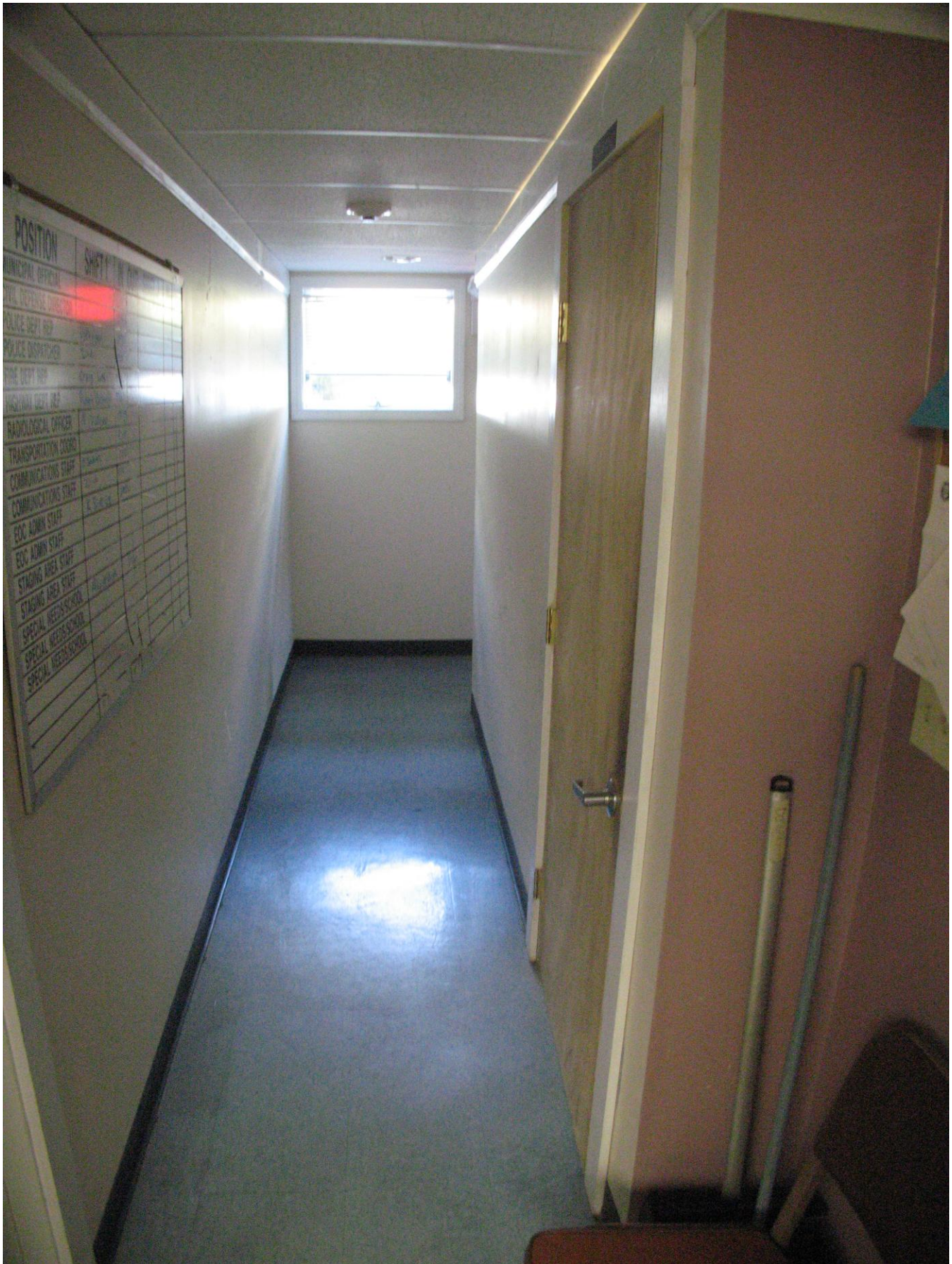
Figure 17: Second means of egress, below minimum requirements
